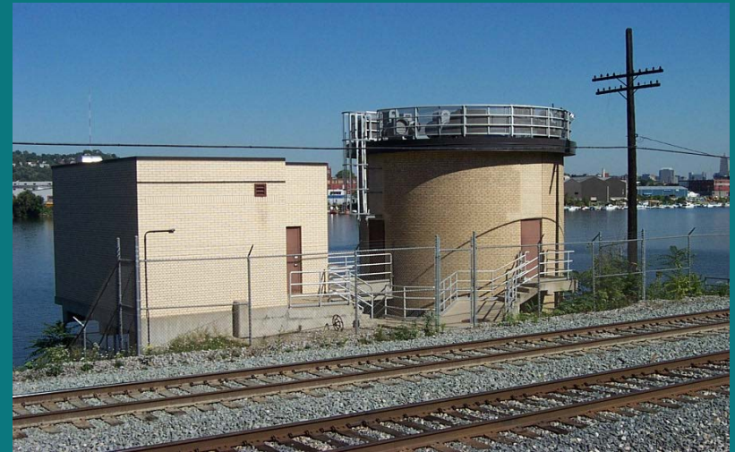
Corliss Pump Station*
