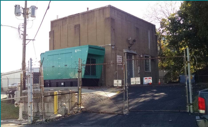
Ella Street Pump Station
