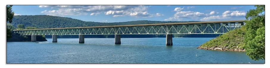
**Bridge Rehabilitation:** SR 59 (Kinzua Road) over the Allegheny Reservoir in Mead Township. Work will include jacking of the bridge superstructure to fix tipped rocker bearings. The bridge is 1,813 feet in length.
